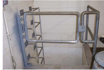
Self-closing swing gate on platform and vertical handrails on ladder Photo courtesy of US Navy.
