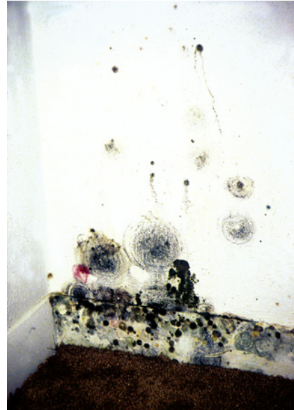
Figure 1: Mold growing on baseboards of a home
