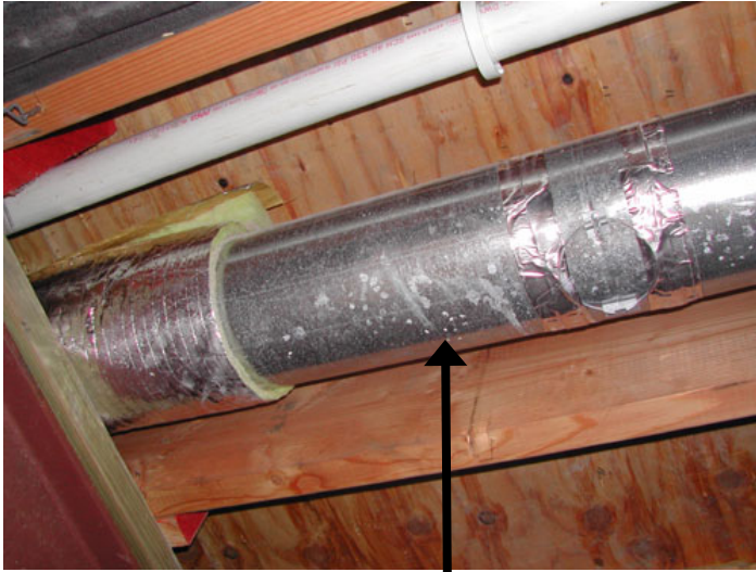
Figure 3: Condensation on pipes
